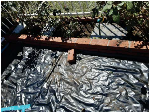
Side Yard Restoration
