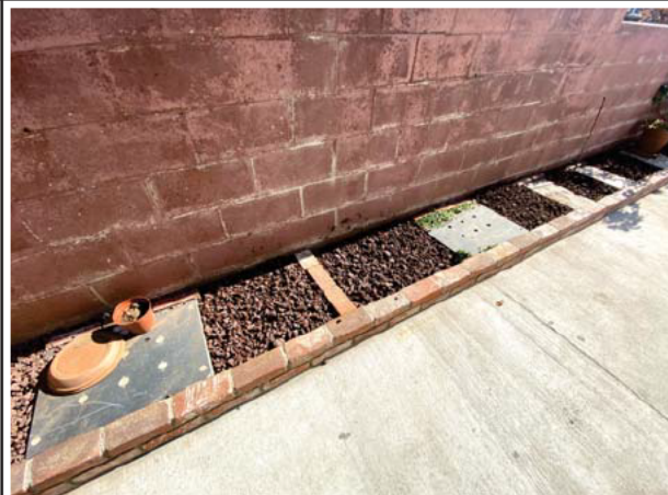
Side Yard Final Restoration
