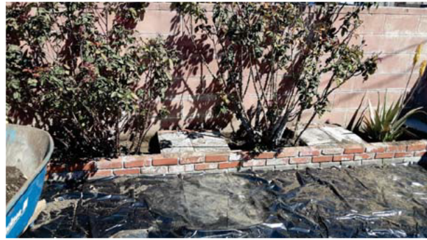
Side Yard Restoration
